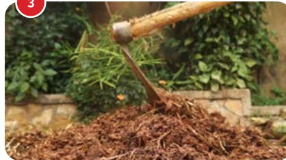
3 Pour water over the soil and grass mixture. Use a hoe to mix until it becomes thick. 1
