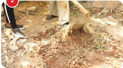
2 Add the dry grass onto the clay soil. Mix evenly using a hoe.
