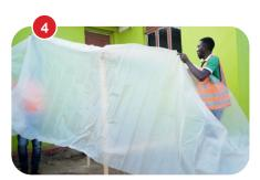
Wrap the frame with a polycarbonate sheet
