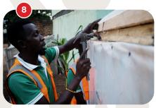
Connect the door to the dryer using door hinges.
