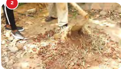
2 Add the dry grass onto the clay soil. Mix evenly using a hoe.
